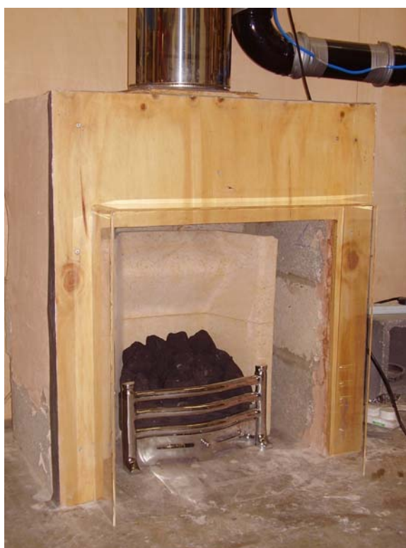
Figure 4 Installation of DFE fire
