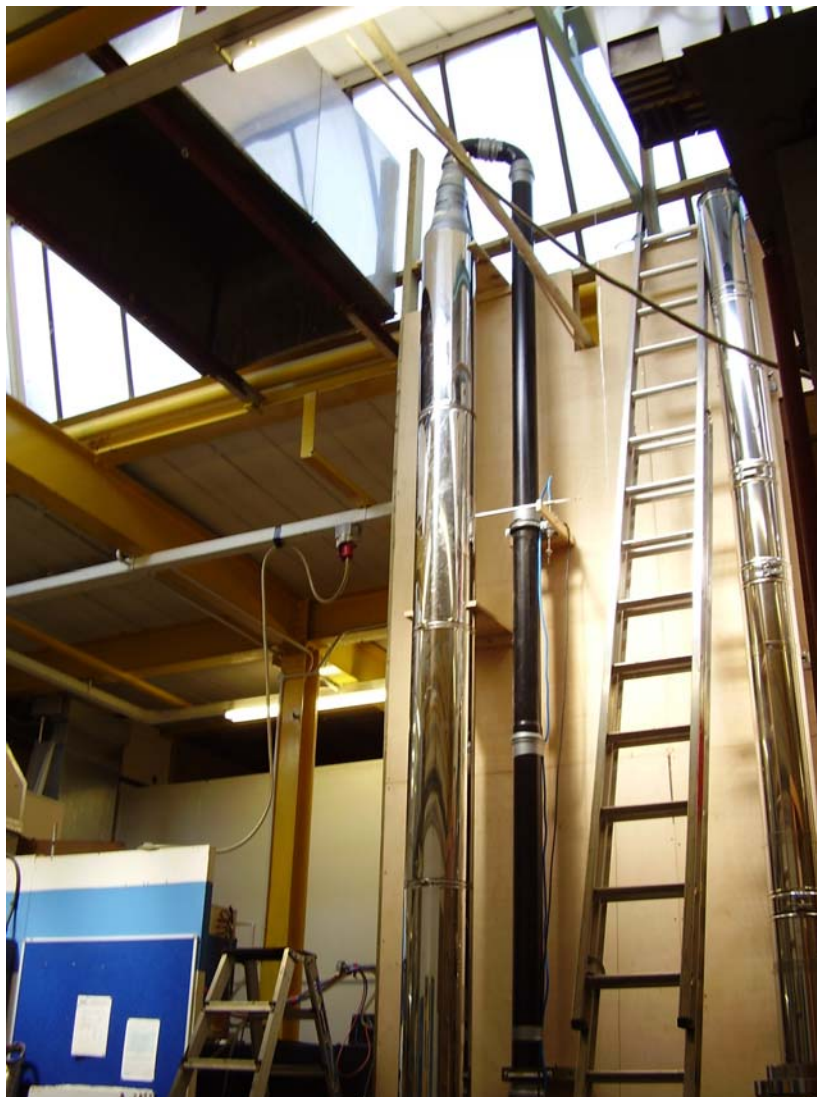
Figure 2 Installation of 200 mm twin wall chimney and air flow measuring system
